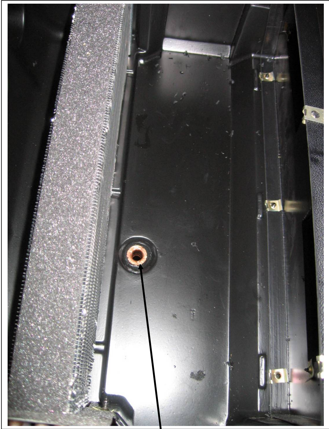
Copper glue in drain tube adaptor in place.
